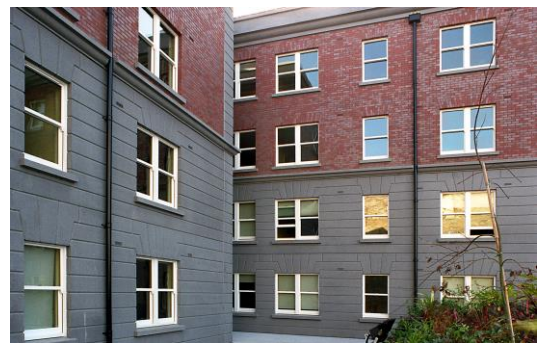
Traditional Sliding Sash Windows Supply and Installation
